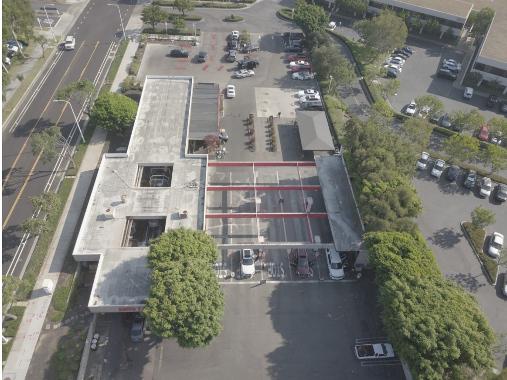
Figure 7: Aerial view of Beacon Bay Auto Wash from northern edge of Project boundary, view south.
