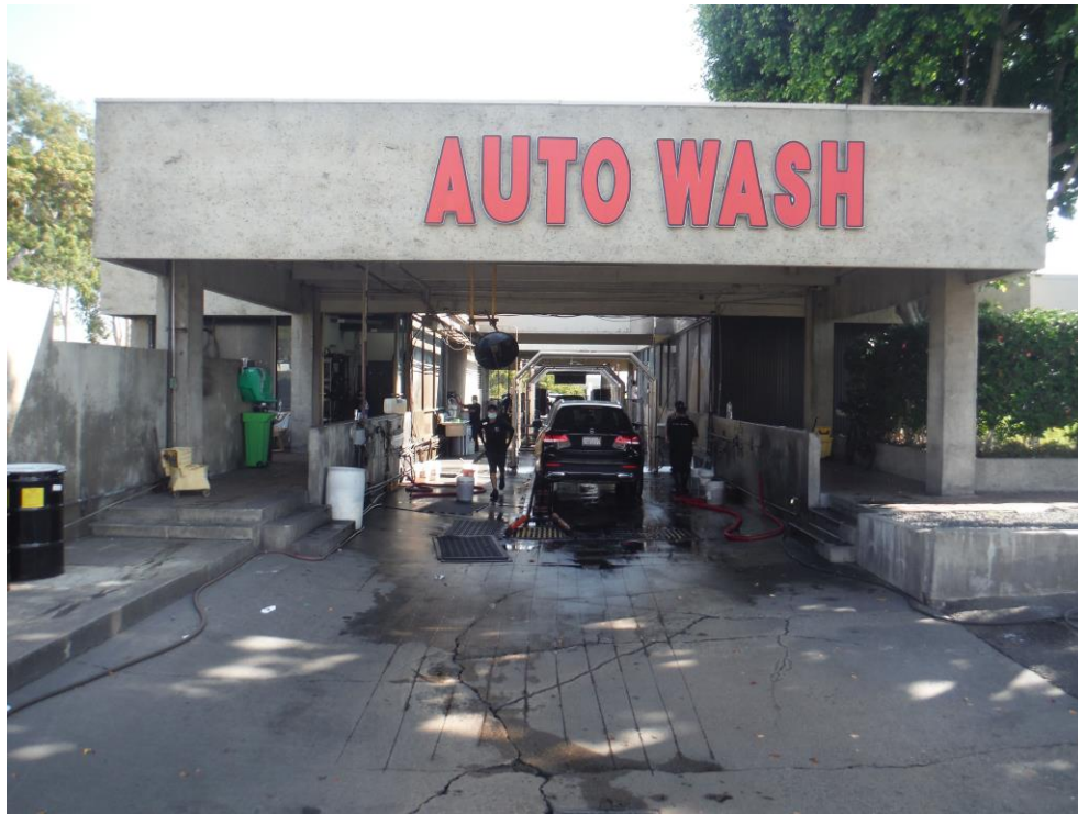
Photograph 9: View of the Auto Wash portion of the facility.
