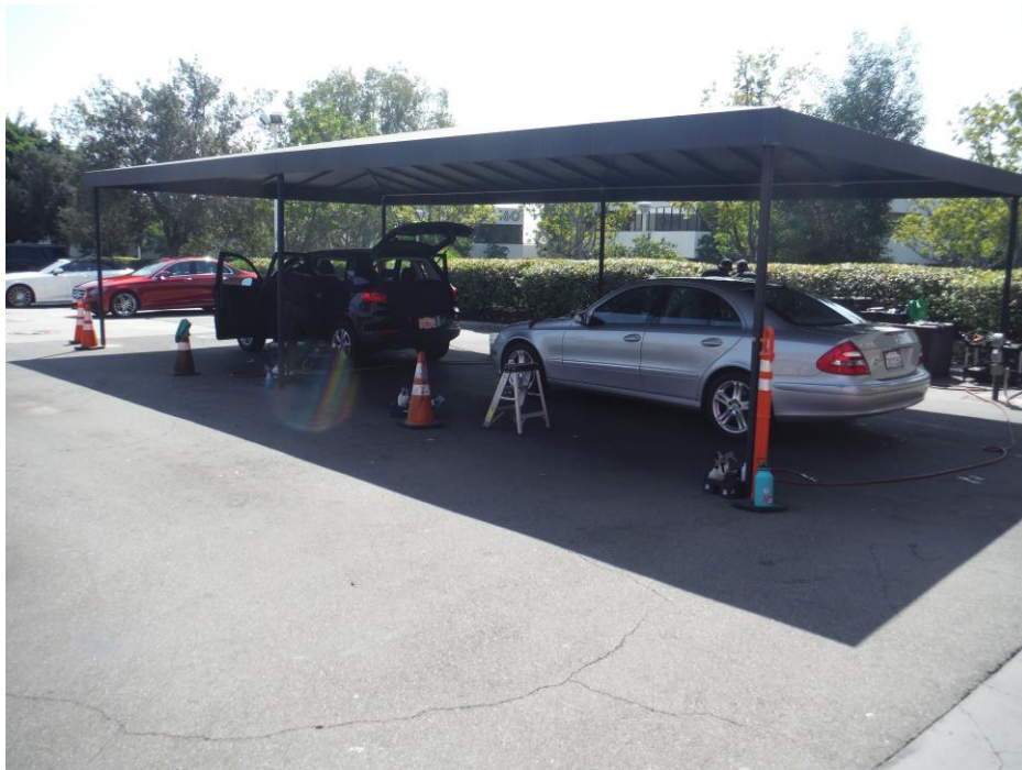
Photograph 6: View of the aluminum detail canopy on the west side of the facility.
