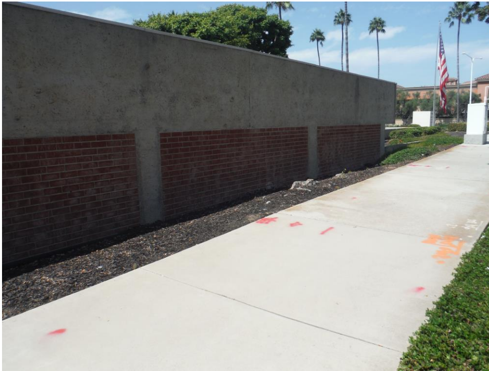
Photograph 3: View looking north at exterior wall detail fronting Anacapa Drive.
