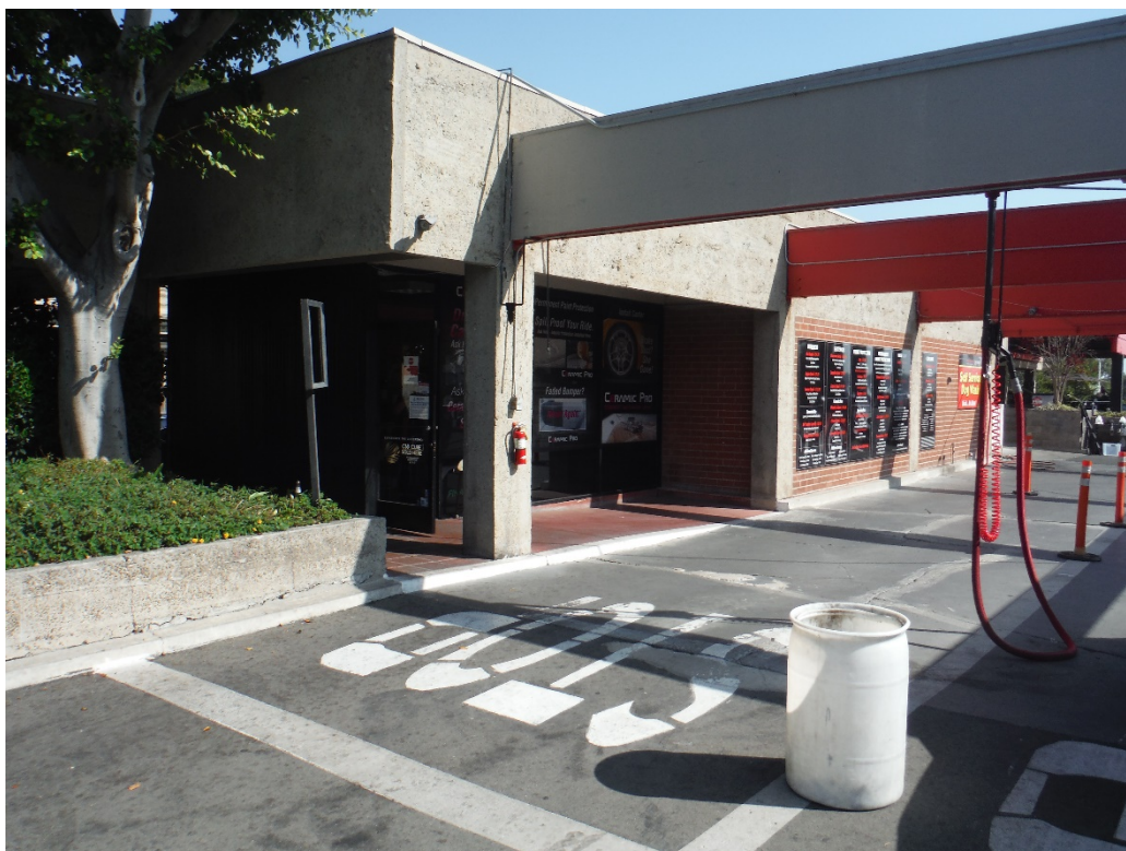
Figure 6: Overview of main building from northern edge of Project boundary, view southeast.
