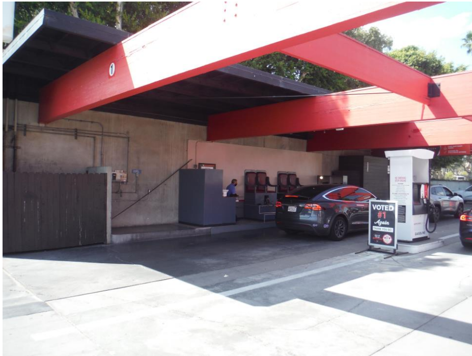
Photograph 7: View of the auto detailing station in the center of the facility, characterized by the large beams or trusswork that connect the western concrete wall to the opposite side of the auto wash on the upper walls of the main office (Photograph 8).
